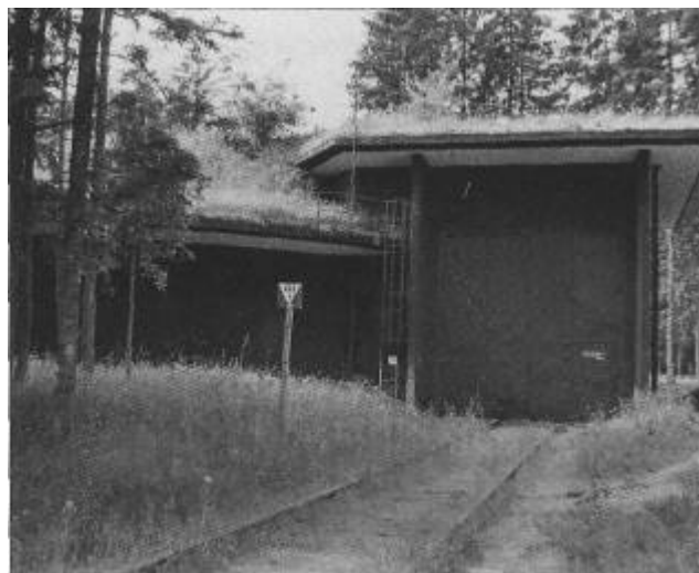
Above: The sinister facade of a German mustard gas storage building, in which the agent was kept in huge concrete vats.
